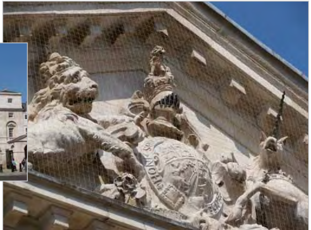
Horse Guard Parade - installed by Beaver Pest Control, London
